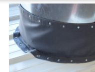
Stretch lower edge to follow profile. Apply construction grade sealant, appropriate for material surface, along bottom edge and fix in valleys
