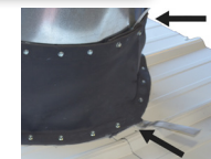
Seal joint by threading metal strip under overlapping joints, starting at the bottom
