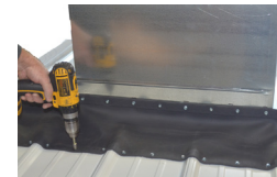
Fasten in valleys and rib corners as shown
