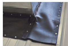
Cut away excess and overlap neatly
