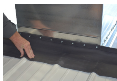
Stretch bottom edge by HAND to follow profile. DO NOT USE TOOLS
