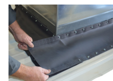
At corners, stretch top edge of each overlap and pull down, then fasten top corner
