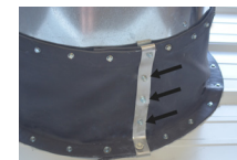
Finish fastening using rivets to bring aluminum pieces together
