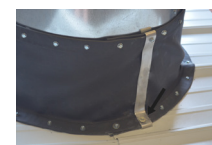
Fasten top edge. Remove and replace bottom screw after forming
